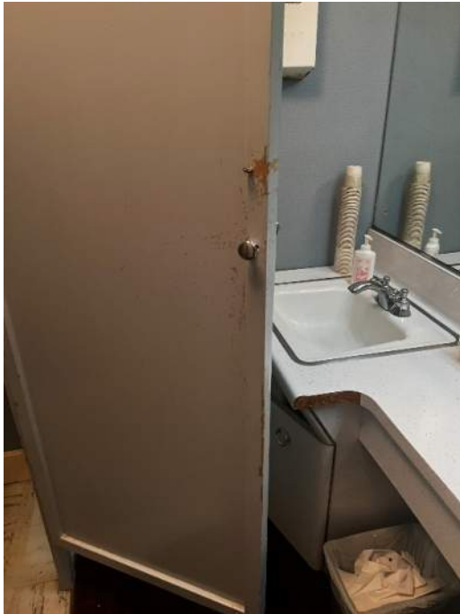
Photo 51: IMG_1441 – Second Floor Gender-Neutral Toilet Room - Toilet room is not ADA compliant or sized adequately for conversion for ADA compliance. Toilet room contains asbestos containing materials (ACM) which require to be abated.
