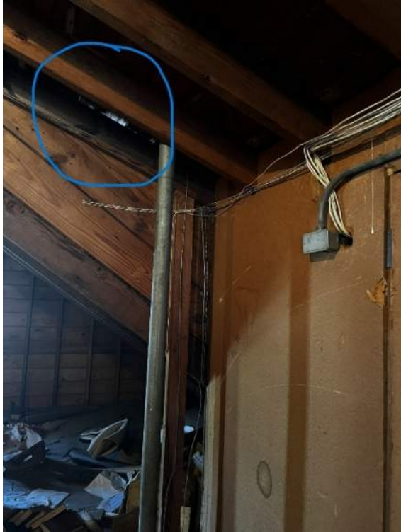
Photo 75: IMG_1579 – Light is visible from below roof framing to exterior.
