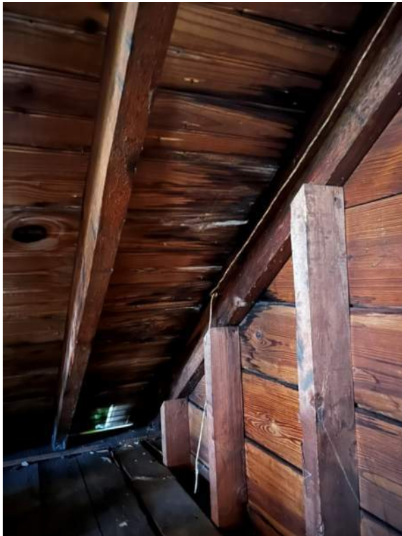
Photo 86: IMG_1563 – Visible water infiltration and moisture damage to roof decking and gable end wall.
