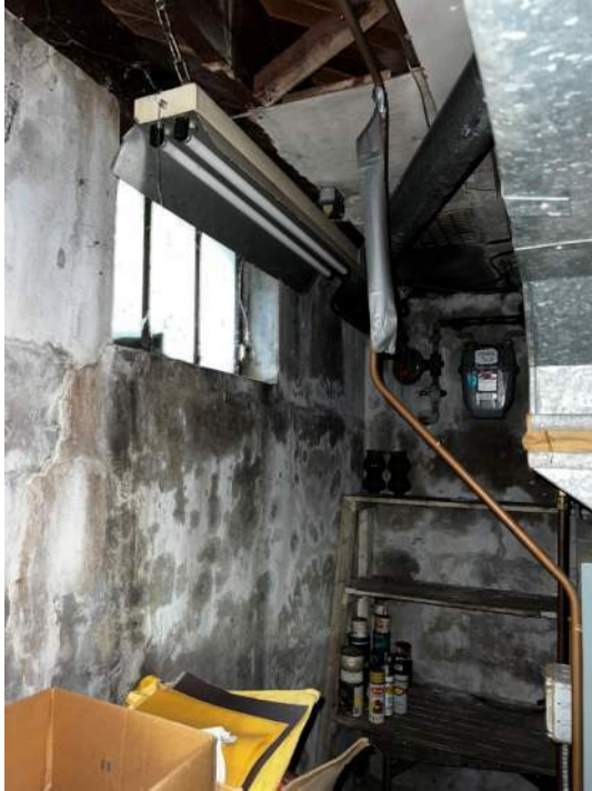
Photo 91: IMG_1251– Significant moisture and water staining is present on Northeast foundation walls.
