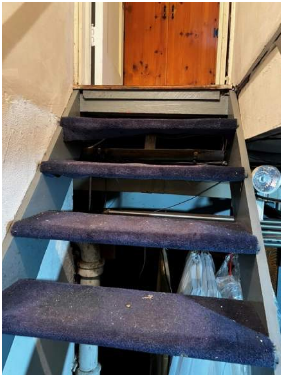
Photo 88: IMG_1244 – Basement egress stairs non-compliant with 2020 BCNYS and are not ADA compliant. Stairs feature non-complaint handrails, open stair treads, and are not enclosed with an exit at an exit discharge or to a public way.
