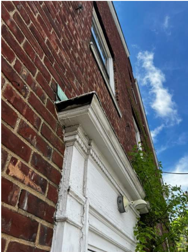
PHOTO 12: IMG_1049 – East Façade – deterioration of wood trim and missing pieces.
