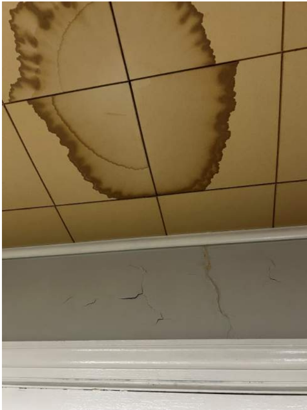
Photo 32: IMG_1197 - Interior 1 st Floor, Anteroom to Prep Room – Visible water damage to ceiling started infiltrating wall.
