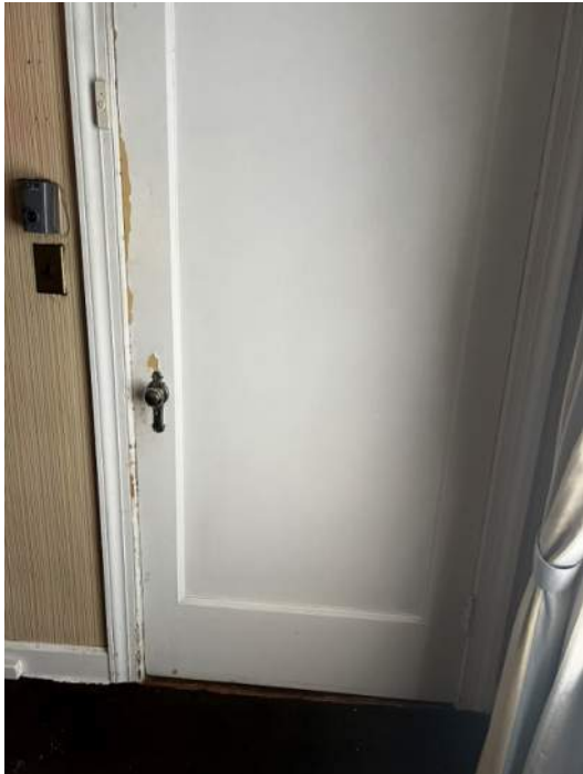
Photo 66: IMG_1502 – Second Floor Southwest Chapel – Elevator shaft enclosure (wall construction and door) are not rated. Per 2020 BCNYS shaft enclosures shall have a fire-resistance rating of not less than 2-hours where connecting four or more stories. This shaft enclosure connects 4-stories (basement, first floor, second floor and attic).
