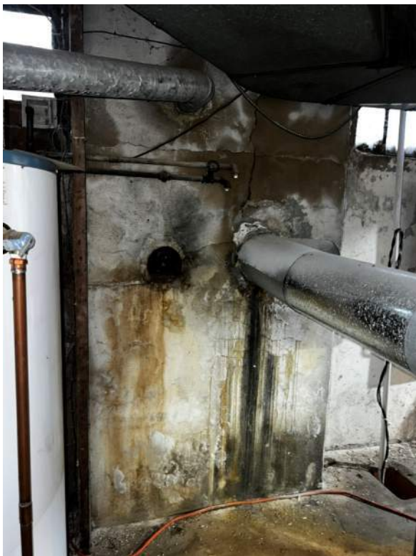
Photo 92: IMG_1256– Significant water damage and staining is present on interior side of East chimney foundation. Foundation for chimney is spalling and contains major vertical and horizontal cracking
