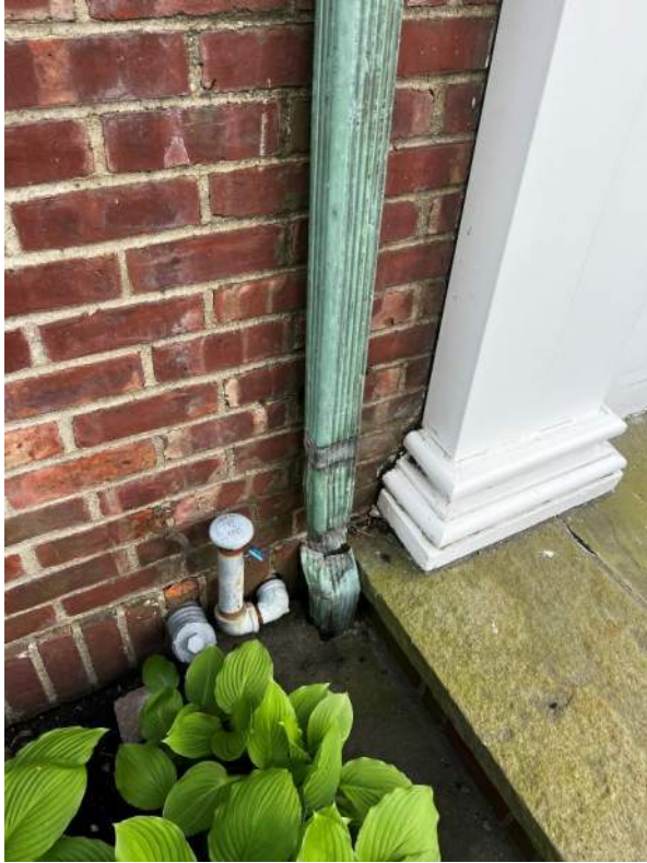
PHOTO 15: IMG_1147 – North Façade – Damaged downspout, allowing water to drain directly to foundation wall.
