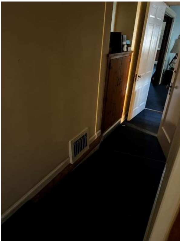
Photo 36: IMG_1208 - Interior 1 st Floor, Hallway from Office to North East room – Floor surface contains a non-compliant ramp – non-compliant slope and no handrails.
