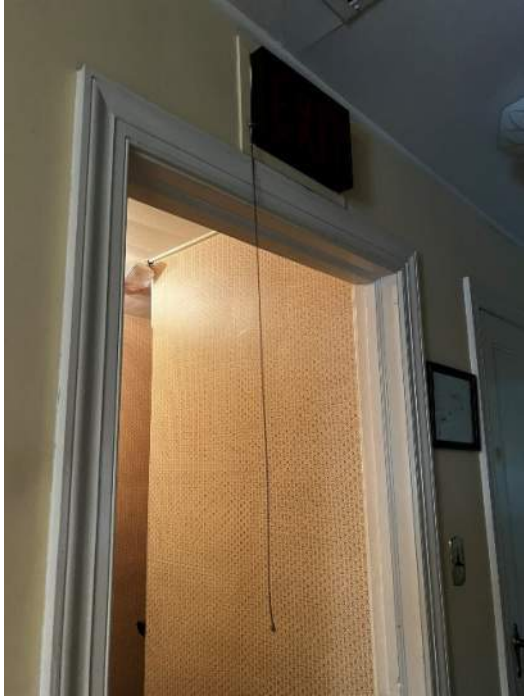
Photo 53: IMG_1445 – Second Floor Corridor – Emergency exit sign is present, but not continuously illuminated. Pull string cord activates illumination. Exit sign is not directional.
