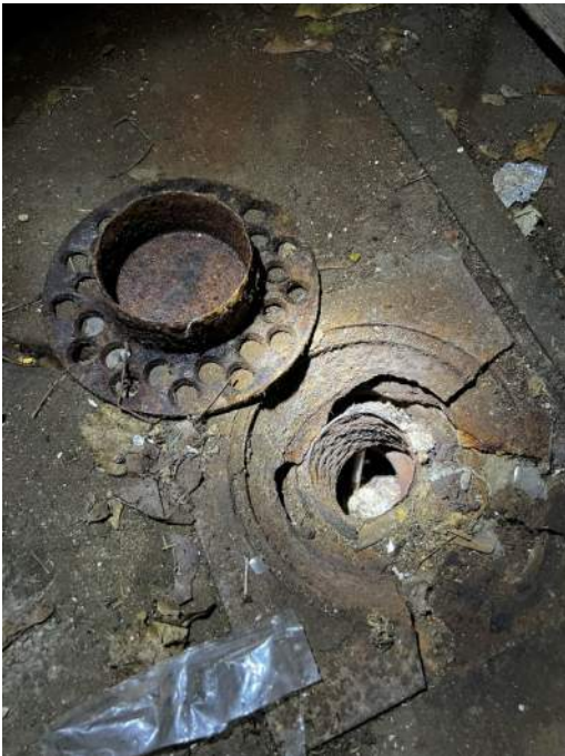
PHOTO 16: IMG_1046 – Clogged floor drains.
