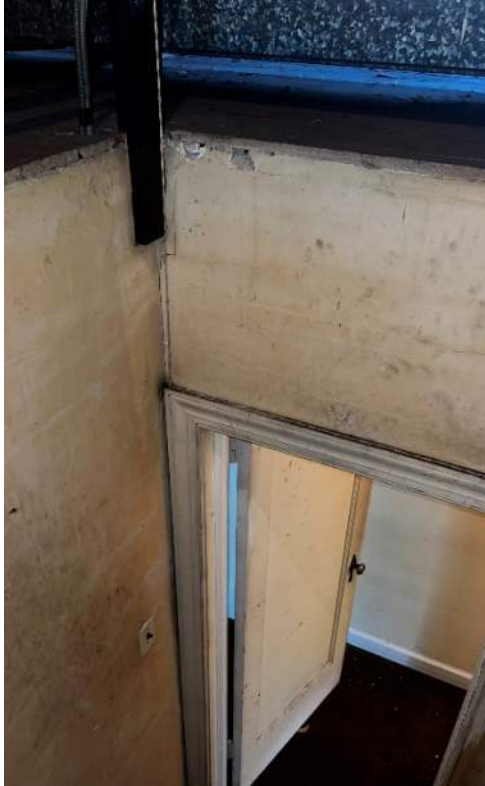
Photo 73: IMG_1535 - Plaster walls on wood-stud wall construction up to attic level. Plaster beginning to crack and degrade, exposing wall cavities.
