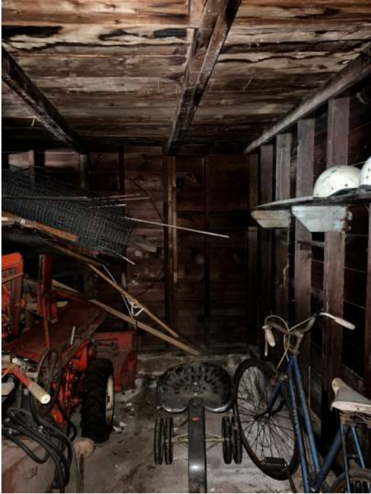
PHOTO 15: IMG_1046 – Visible staining and water damage at wood roof deck.
