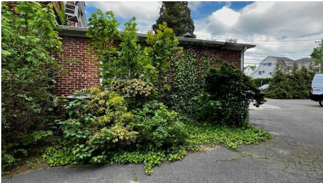
PHOTO 20: IMG_1320 – West Facade–Significant ivy growth which should be removed.
