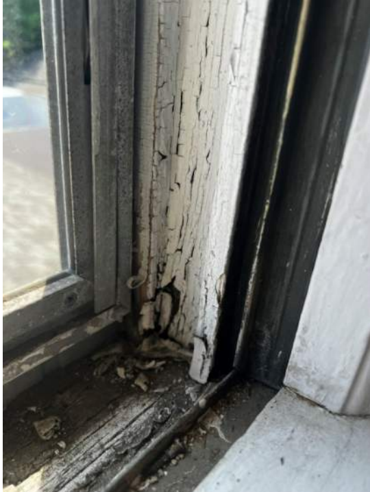
Photo 47: IMG_1435 - East side egress stair, top landing – Window is operable. Interior jambs of window are exhibiting deterioration of paint finish and wood below. Aluminum storm screen can be seen.
