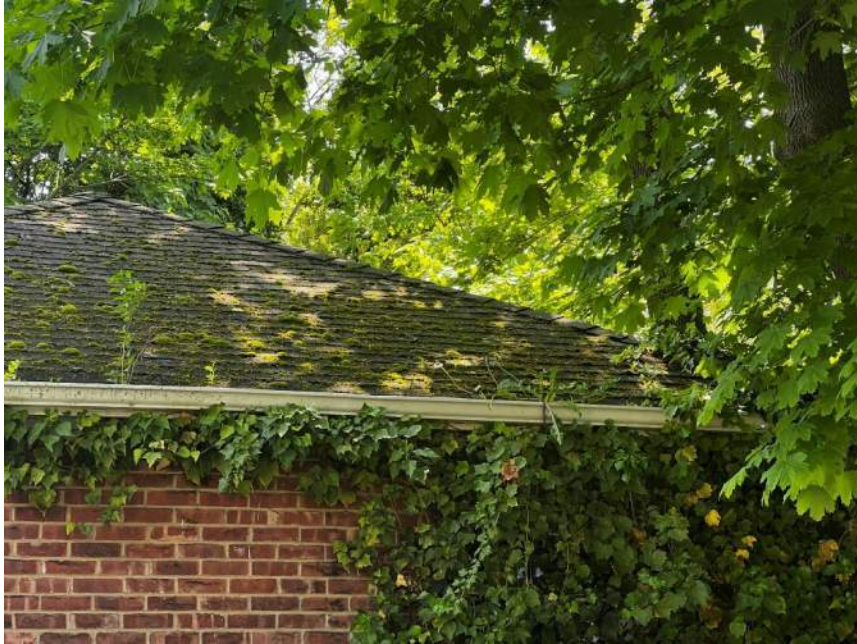
PHOTO 19: IMG_1412 – North Side Roof - Visible moss on roof structure.
