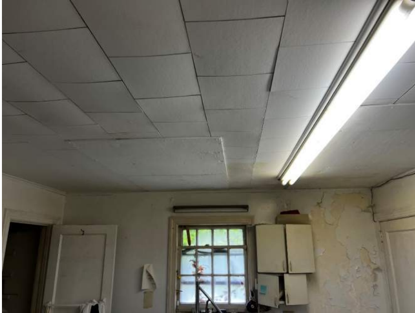
Photo 31: IMG_1191 - Interior 1 st Floor, Prep Room – Prep Room ceiling exhibits visible sagging with patching (Photo 31). Evident ponding on roof above and surrounding areas infers water infiltration issues (photo 68).
