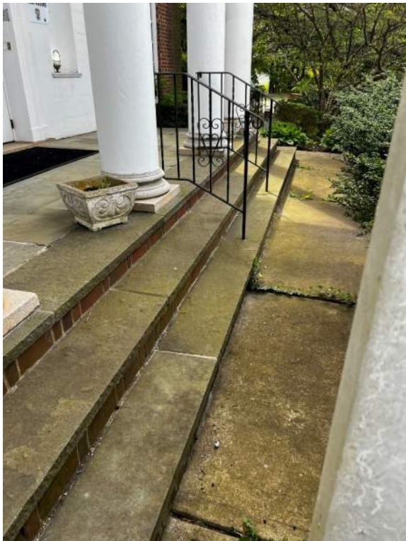
PHOTO 14: IMG_1156 – North Façade – Main entrance and acting egress door exits is not ADA accessible. Non-compliant handrails, riser and tread heights, and does not contain a ramp.
