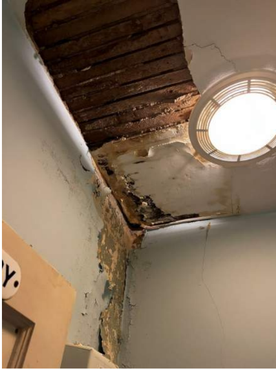
Photo 33: IMG_1207 - Interior 1 st Floor, Gender Neutral Lavatory (North) – Water damage has caused significant ceiling disintegration and damage to original lath and plaster ceiling.
