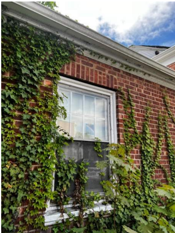
PHOTO 8: IMG_1106 – East Façade – Ivy Growth on walls and gutters, rusted lintels, single pane glazing, wood sills and frame.
