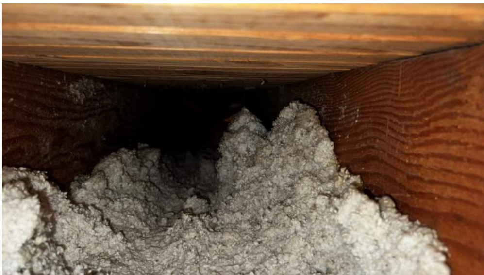
Photo 72: IMG_1534 – Non-compliant loose fill insulation per 2020 ECCNYS between 2x10 floor joists. Insulation values are not marked.
