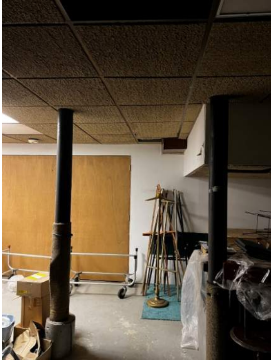
Photo 95: IMG_1672– Elevator shaft at Basement Level – Contains non-compliant UL rated assembly for 2-hour enclosure, typical of 3 doors at basement level. West entrance door into shaft way is a single wood door with wood frame. South entrance door into shaft way is a double wood door with wood frame.
