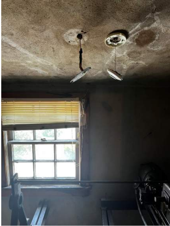
Photo 85: IMG_1588 – Elevator shaftway contains a window. Per 2020 BCNYS shaft enclosures shall have a fire-resistance rating of not less than 2-hours. Window opening requires to have the same fire-rating as the wall assembly. Elevator shaft way contains non-functioning fire alarm devices.
