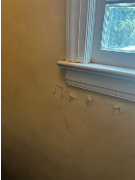
Photo 45: IMG_1430 - East side egress stair, top landing – Plaster wall finish is chipping and peeling from evident water infiltration and moisture into wall finish.
