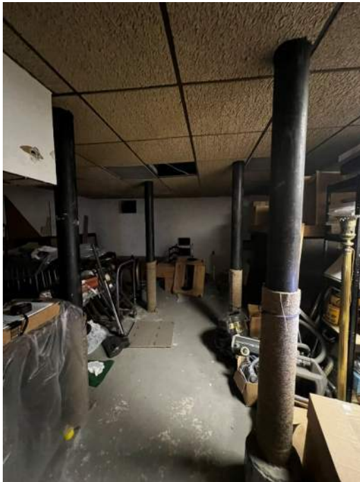
Photo 98: IMG_1669– Basement – South back room (below office) – Contains steel lally columns with non-uniform spacing. Column placement and spacing suggests additional columns were added for reconfiguration of openings on first floor,
