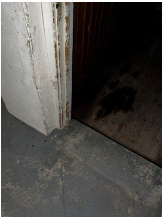
Photo 94: IMG_1651– Elevator shaft at Basement Level – Contains non-compliant UL rated assembly for 2-hour enclosure, typical of 3 doors at basement level. West entrance door into shaftway is a single wood door with wood frame. South entrance door into shaftway is a double wood door with wood frame.
