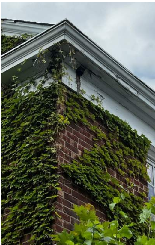
PHOTO 22: IMG_1313 – South Façade - Missing downspout, significant deterioration of wood fascia, rake boards and soffit.
