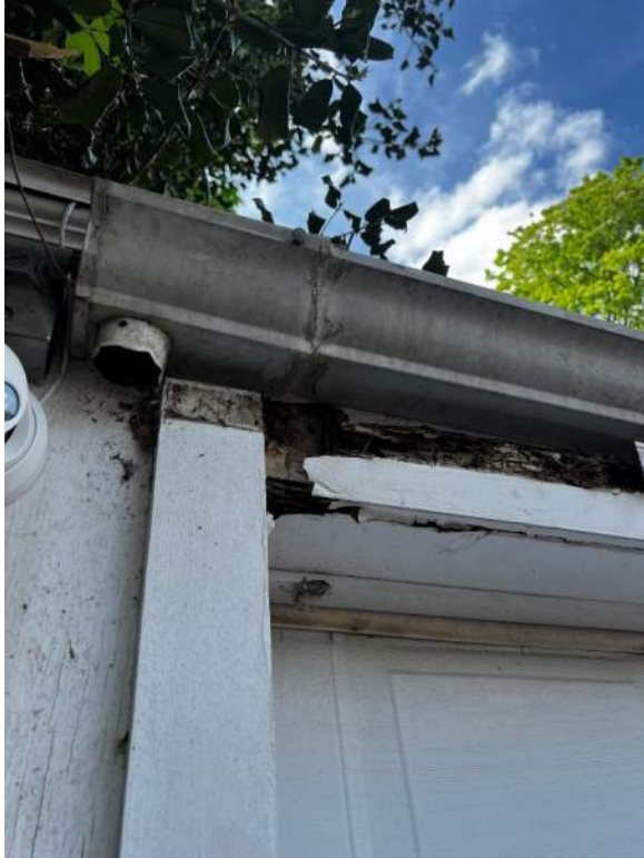
PHOTO 9: IMG_1067 – North Façade. Deteriorated overhead door trim and header. Missing downspouts. Deteriorated seams at gutter.
