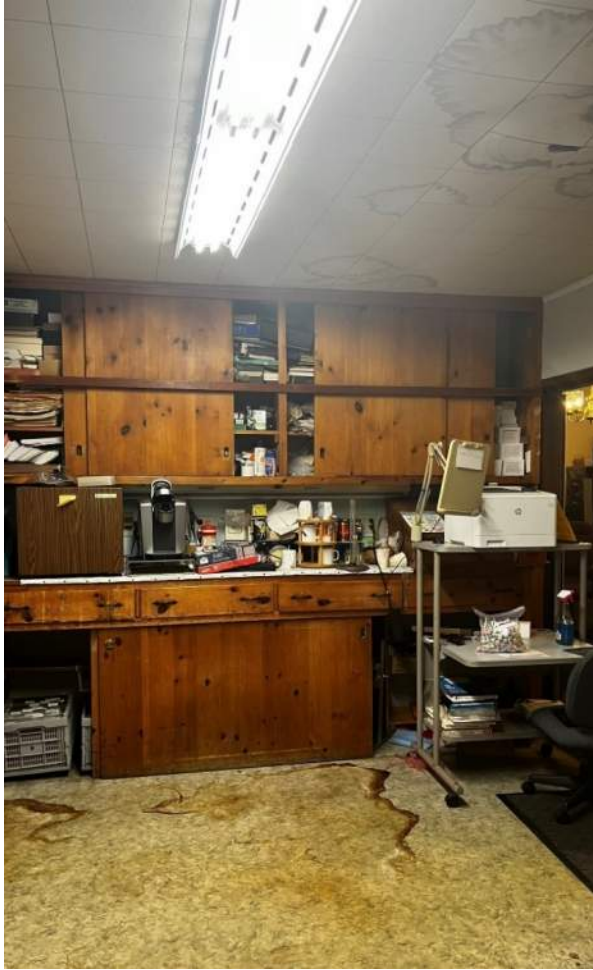
Photo 28: IMG_1426 - Interior 1 st Floor, Anteroom to Prep Room – Significant water damage to the ceiling finish, including ceiling staining, wet ceiling tiles, present puddles and staining at floor.
