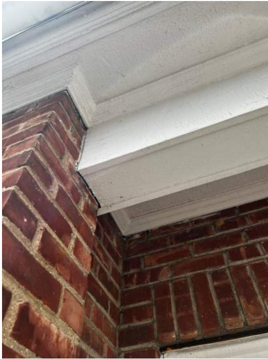
PHOTO 5: IMG_1093 – South Façade – age of wood & visible shrinkage
