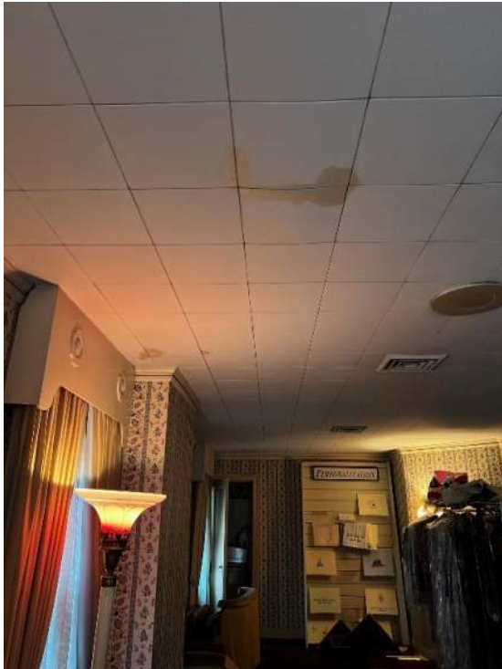
Photo 57: IMG_1466 – Second Floor East Chapel – Visible water damage and active leak at ceiling. Ceiling stain is wet to the touch.
