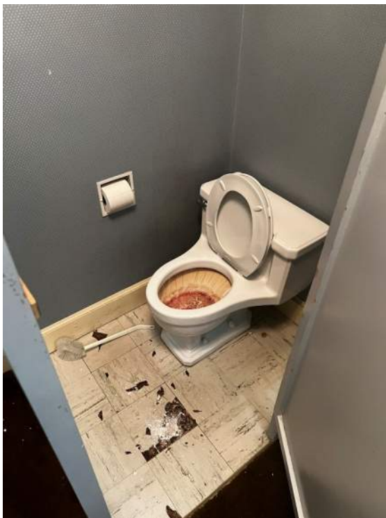
Photo 50: IMG_1440 – Second Floor Gender-Neutral Toilet Room - Toilet room is not ADA compliant or sized adequately for conversion for ADA compliance. Toilet room contains asbestos containing materials (ACM) which require to be abated.
