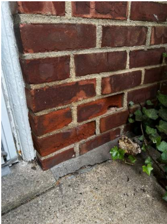
PHOTO 2: IMG_1101 South Façade – Wear on bricks, general staining
