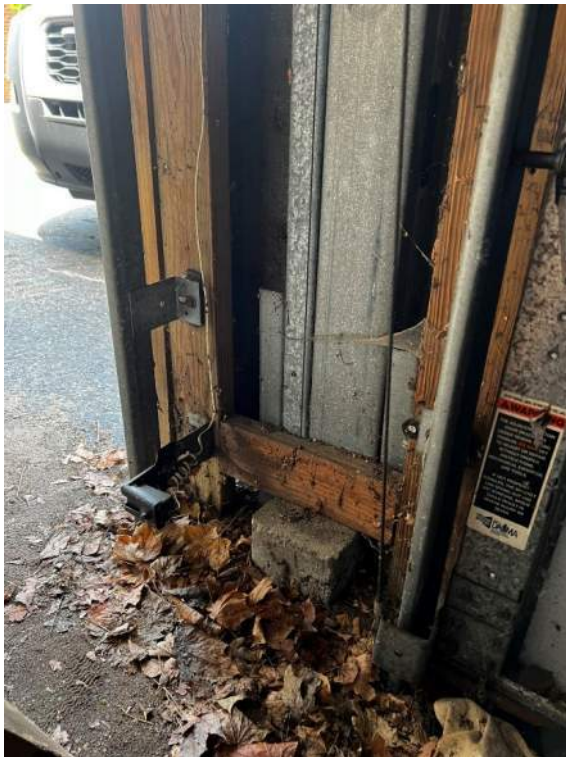
PHOTO 4: IMG_1041 Addition – Metal stud does not rest on built foundation.
