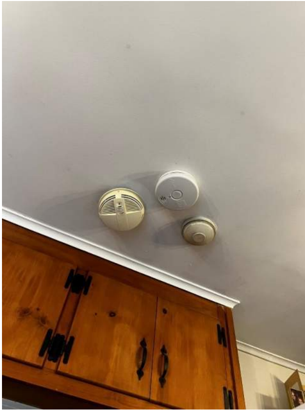
Photo 27: IMG_1173 - Interior 1 st Floor, Rear Office – Multiple fire alarm devices, non-hard wired carbon monoxide detector. Assumed redundant devices due to non-functioning system.
