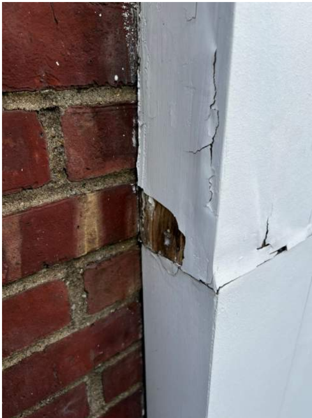
PHOTO 16: IMG_1148 – North Façade – Painted wood façade elements are chipping, exposing the wood to the elements. Wood has begun to weather.
