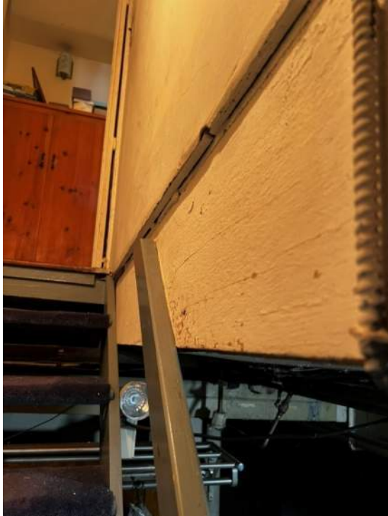
Photo 89: IMG_1243– Basement egress stairs non-compliant with 2020 BCNYS and are not ADA compliant. Stairs feature non-complaint handrails, open stair treads, and are not enclosed with an exit at an exit discharge or to a public way.
