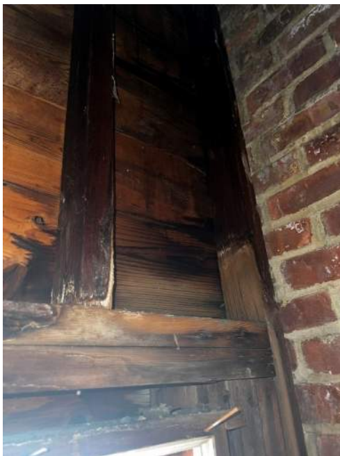
Photo 82: IMG_1557 – Wood framing above windows on East side attic exhibit significant water damage. The visible water damage aligns with the brick bulging (photo 10) from exterior which indicates significant water damage is likely to be found at all window framing on East wall.
