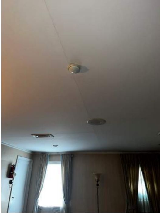
Photo 65: IMG_1497 – Second Floor Southwest Chapel – Ceiling exhibits cracking due to deflection of wood framing. Cracks in ceiling run full length and width of room. Building does not contain emergency egress lights; main source of illumination is portable lamps.
