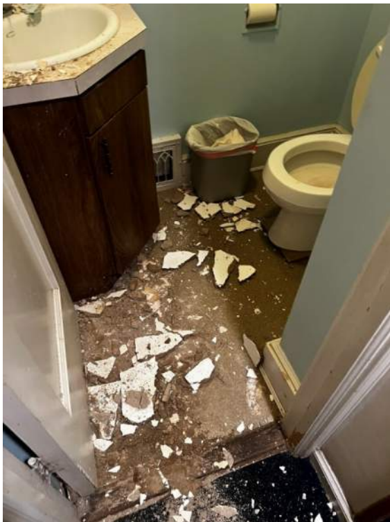
Photo 34: IMG_1205 - Interior 1 st Floor, Gender Neutral Lavatory (North) – Water damage has caused significant ceiling disintegration and damage to original lath and plaster ceiling. Toilet room is not ADA compliant.
