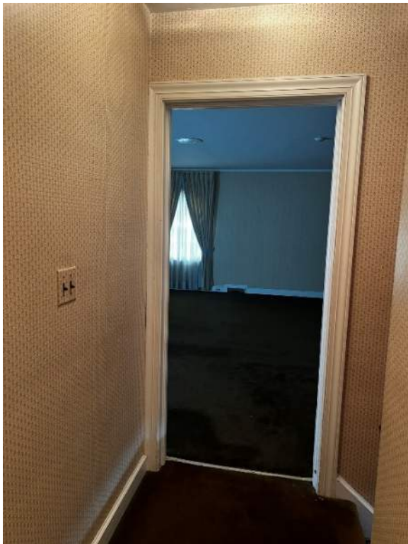
Photo 56: IMG_1459 – Second Floor Landing at Top of Main Stair – Non handicap accessible clearances at doorways and stair landings. Non-compliant handrail extensions.
