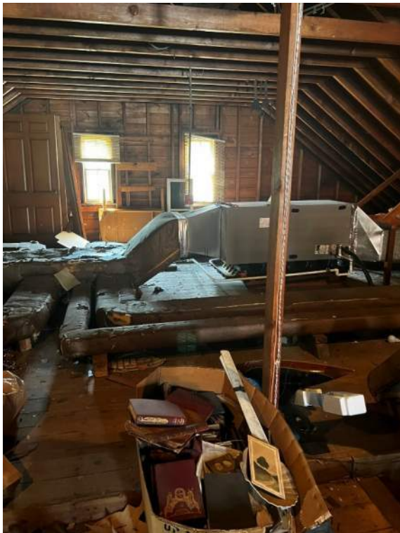
Photo 70: IMG_1597 – Attic appliances – Attic does not contain a clear passageway for removal of the largest appliance; passageway is obstructed by ductwork and dunnage.
