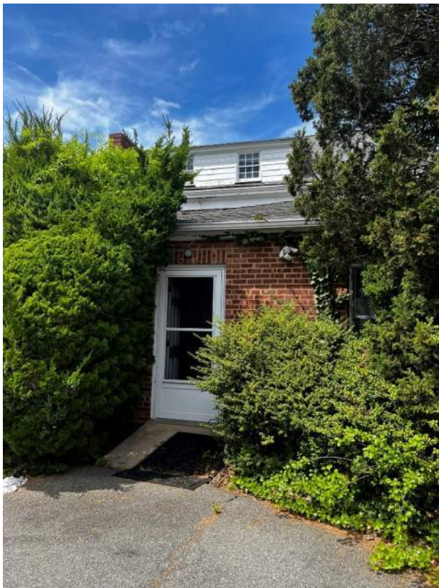
PHOTO 6: IMG_1104 – South Façade – Non-compliant ADA ramp top door, door swings in, rusting lintels.
