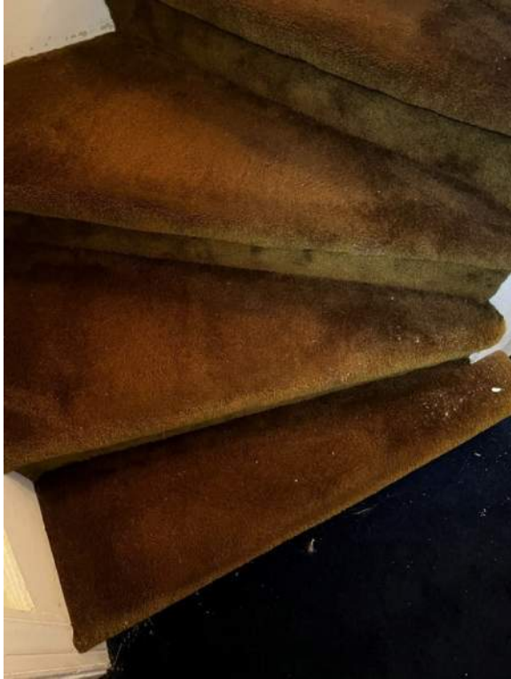
Photo 41: IMG_1237 - Interior 1 st Floor East side egress stair – Contains winder treads.
