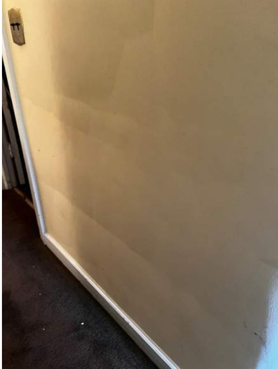
Photo 55: IMG_1449 – Second Floor Corridor – Plaster wall finish is uneven, bowing and bulging.
