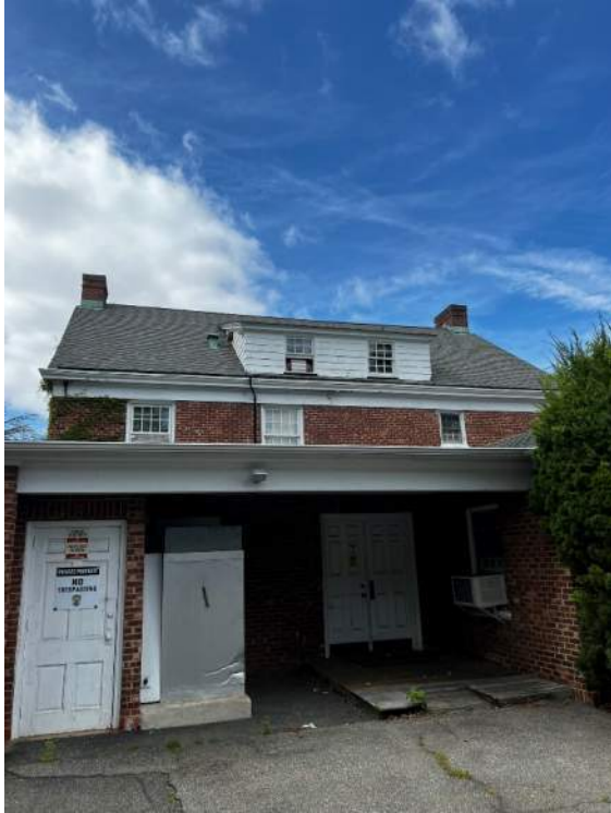
Photo 25: IMG_1351 - South Facade – No visible flashing from reverse gable roof to second story brick masonry wall. Damage to cedar shake at attic dormer.
