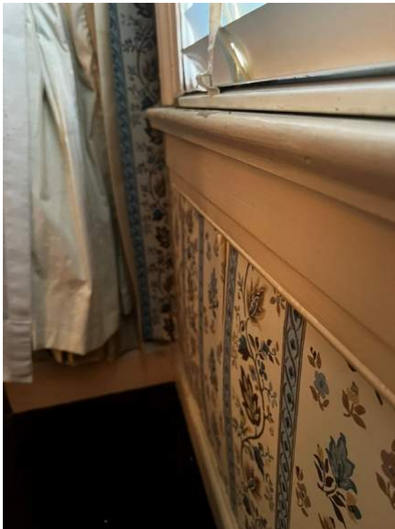
Photo 60: IMG_1476 – Second Floor East Chapel – Walls below East windows exhibiting bowing due to water infiltration.
