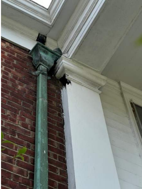
PHOTO 17: IMG_1151 – North Façade (North East of front entrance) - Internal downspout to collector box is dislodged, allowing water to drain onto brick masonry and wooden elements.
