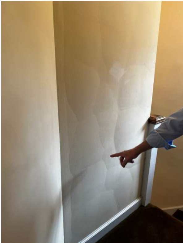
Photo 54: IMG_1446 – Second Floor Corridor – Plaster wall finish is uneven, bowing and bulging.
