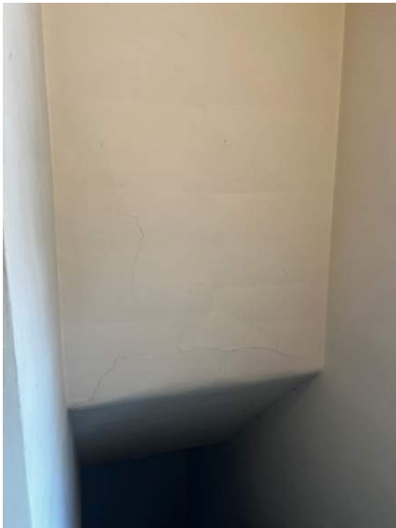
Photo 46: IMG_1428 - East side egress stair, top landing – Plaster wall finish beginning to crack, bulge and bow at area above stairs. Requires refinishing.
