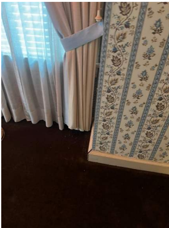
Photo 58: IMG_1473 – Second Floor East Chapel – Chimney exhibits visible bowing with subsequent damage to the baseboard trim from the masonry movement.
