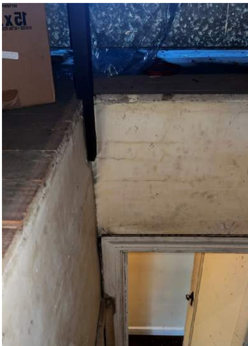
Photo 74: IMG_1536 - Stairs do not contain code compliant balustrades, guards or adequate opening limitations that would prevent the passage of a 4" sphere.
