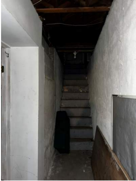
Photo 97: IMG_1276– Basement stairs to Exterior – Non-compliant riser and tread heights per 2020 BCNYS 1011.5.2. Existing poured concrete stairs have a 9.5” riser height and a 9.25” tread depth. Stairs do not contain handrails. Landing at top of stairs is not compliant with 2020 BCNYS 1012.6.3 the landing length shall be 60 inches minimum. Approach to door is not ADA compliant.
