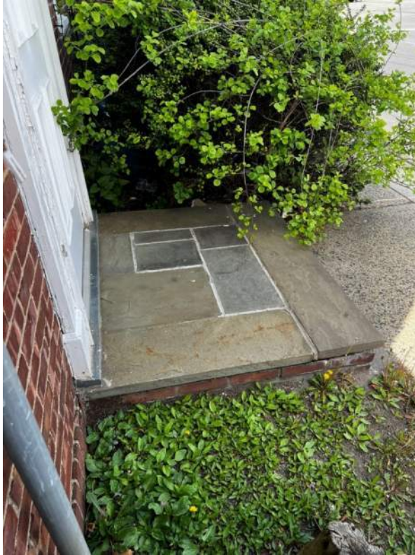
PHOTO 13: IMG_1017 – East Façade – Emergency exit door with non-compliant landing/elevation.
