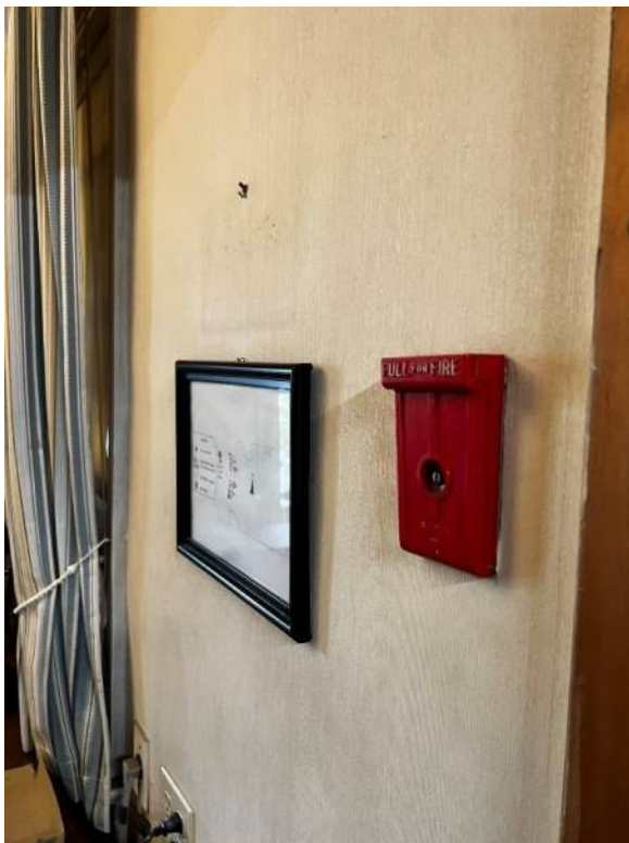
Photo 26: IMG_1170 - Interior 1 st Floor, Rear Office – Non-functioning pull stations.
