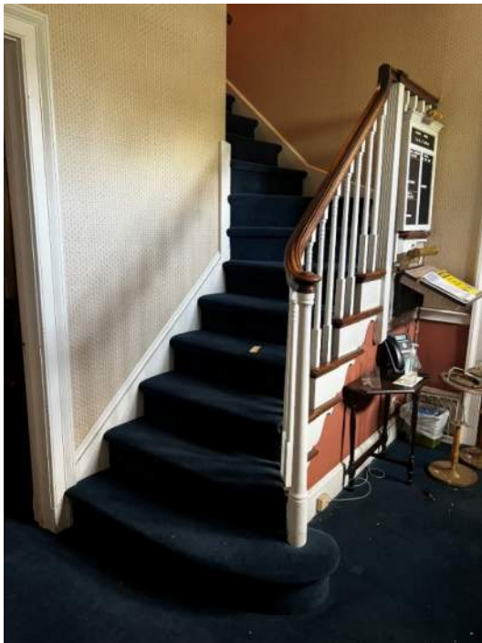
Photo 38: IMG_1220 - Interior 1 st Floor, Main Stair is non-compliant with 2020 BCNYS Chapter 10 Means of Egress Sizing : 2'-10 ½" clear width, 2'-7" High handrail height, 3'-3 ½" guardrail height and winder stair treads. Handrails are not continuous without interruption by newel posts and do not extend past the top and bottom risers (2020 BCNYS 1012.4 & 1012.5). Handrails are not present on each side (2020 BCNYS 1009.10).
