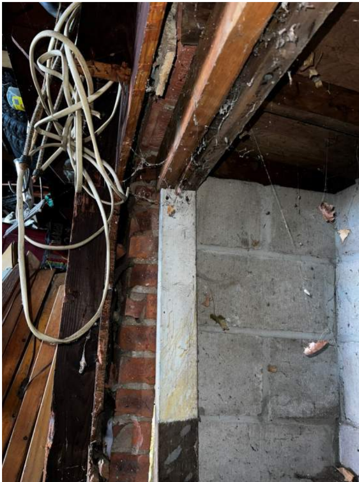
PHOTO 18: IMG_1029 – Brick is not properly supported from below at opening. Horizontal wood member supports the framing of the roof over the CMU bump-out.
