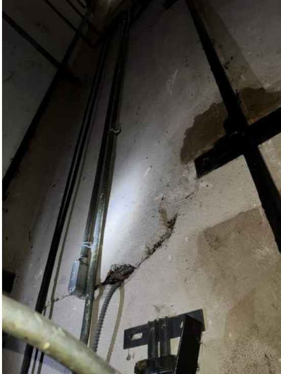
Photo 93: IMG_1251– Elevator shaft at Basement Level – Contains significant cracks and pipe penetrations that are not sealed as required for 2-hr fire rating at shaft way.
