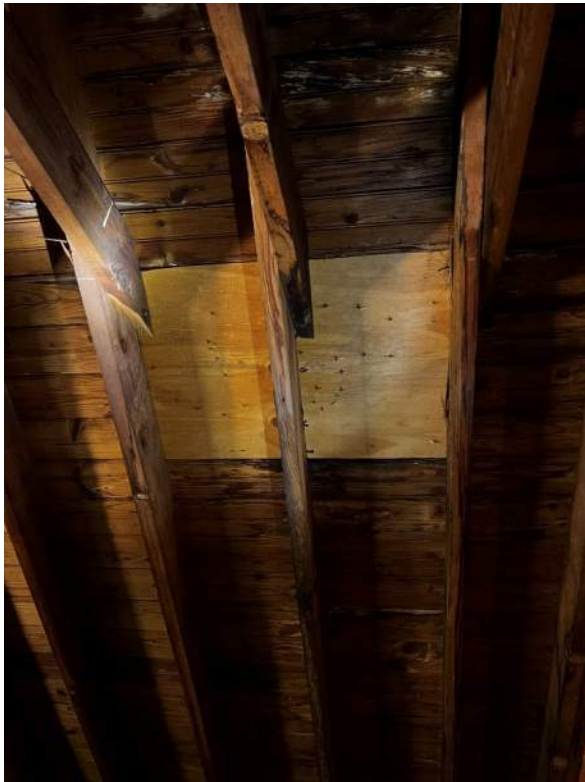
Photo 80: IMG_1577 – Roof Deck – Areas of roof deck have been replaced. Review of asphalt shingle roof is recommended.
