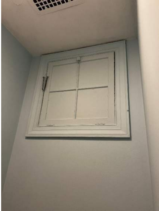
Photo 35: IMG_1208 - Interior 1 st Floor, Gender Neutral Lavatory (North) – Operable window opens to interior framing. Indicates possible reconstruction or additions of existing building.
