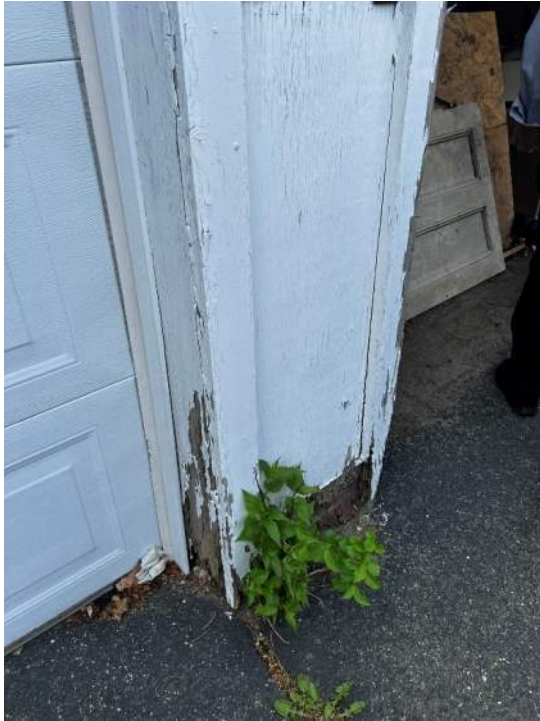
PHOTO 4: IMG_1012 Addition – Exterior wall finish deterioration
