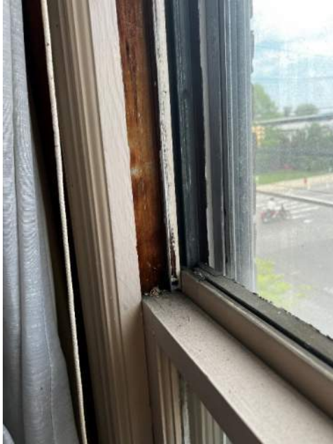
Photo 43: IMG_1468 - Interior 2 nd Floor, East Funeral Chapel (& throughout) – Various windows are non-functional throughout entire building. The windows throughout utilize a rope and pulley string for operation; various windows contain ropes that have dry-rotted and subsequently, broken. Many windows with rope and pulley systems intact are non-functional due to multiple layers of paint and lack of use leaving a handful of windows operable for ventilation purposes.
