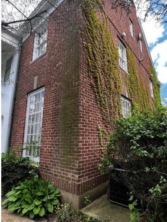
PHOTO 19: IMG_1325 – North West Corner – Significant mold and mildew on North Façade. Significant ivy growth which should be removed on West facade.
