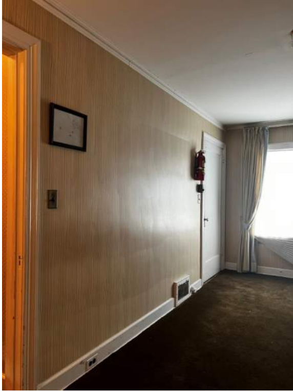
Photo 67: IMG_1507 – Second Floor Southwest Chapel – Wall finish exhibits bowing at interior walls. Fire extinguisher is not mounted in compliance with NFPA 10. Light switches and receptacles are not mounted in compliance with ADA.
