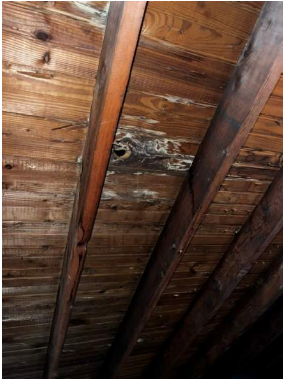
Photo 81: IMG_1601 – Roof Deck – Visible rot and moisture infiltration at roof deck in Northeast portion of attic.
