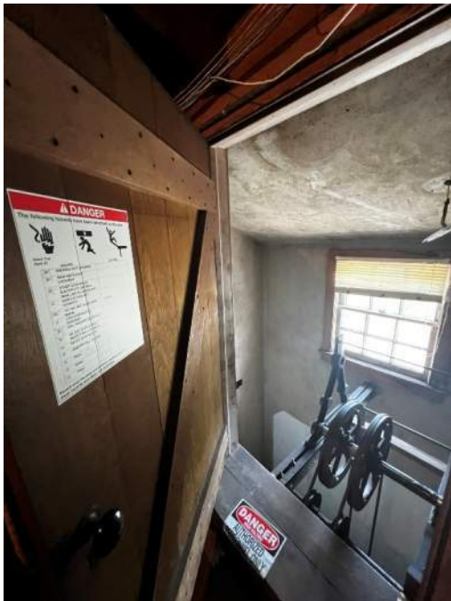
Photo 84: IMG_1584 – Elevator access door opens to elevator shaft way with no fall protection. Per OSHA 1917.116, elevator landing openings shall be provided with doors, gates or equivalent protection which shall be in place when the elevator is not at that landing, to prevent employees from falling into the shaft.
