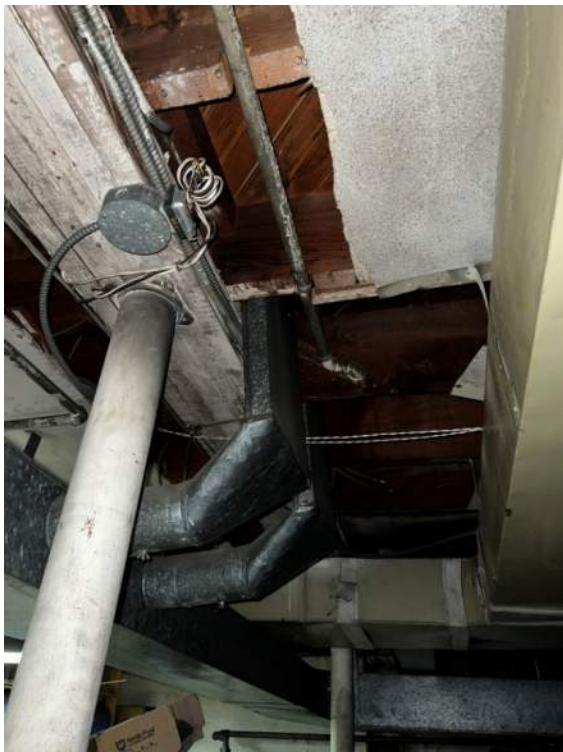
Photo 90: IMG_1248– Floor joists feature notches and holes. If configuration of interior walls, stairwells, finishes are altered and changing structural dead loads, and if interior live loads are altered based on occupancy reclassification, joists shall require to be evaluated by a structural engineer.
