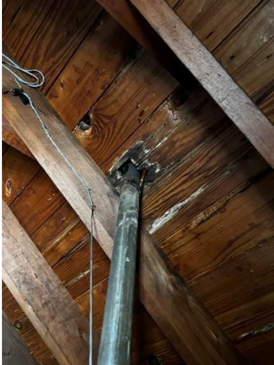
Photo 79: IMG_1576 – Roof Deck – Visible rot and moisture infiltration at roof deck surrounding plumbing vent stack indicating inadequate flashing.
