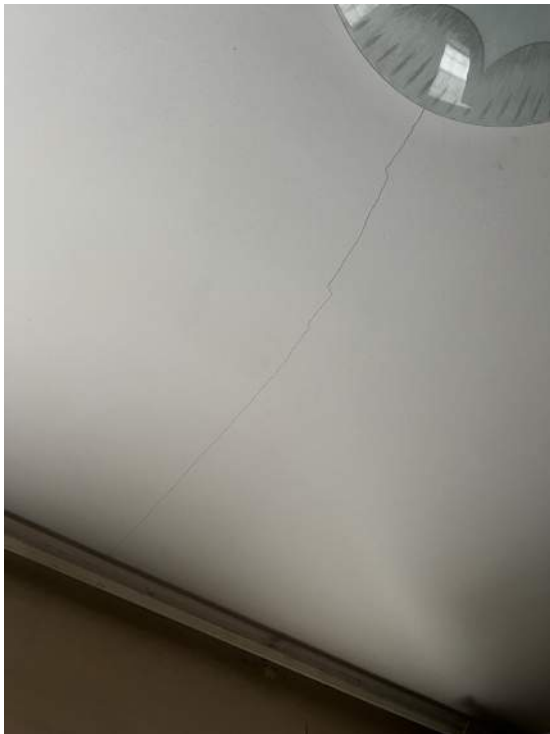
Photo 62: IMG_1489 – Second Floor North Anteroom – Ceiling exhibits cracking due to deflection of wood framing.
