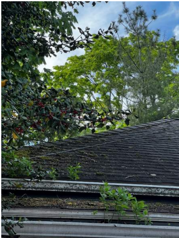
PHOTO 14: IMG_1082 – East Side Roof - Visible moss on roof structure.
