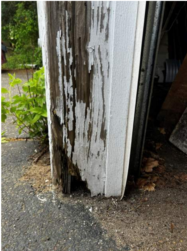
PHOTO 10: IMG_1067 – North Façade. Deteriorated overhead door jambs.
