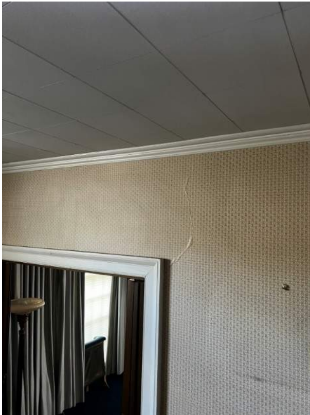
Photo 40: IMG_1224 - Interior 1 st Floor Main Entrance – Wall cracking is present below wallcovering finish.
