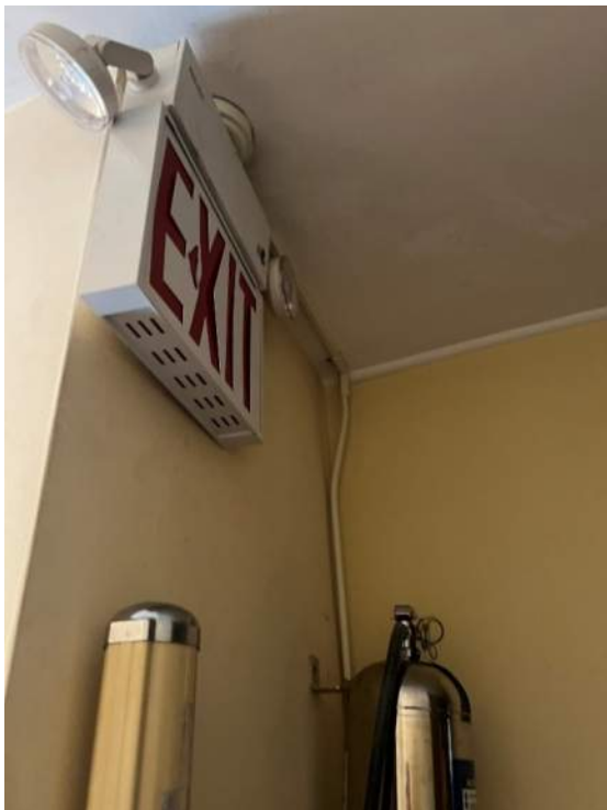
Photo 48: IMG_1438 – Second Floor Hallway to East side egress stair. Emergency exit sign is present, but not continuously illuminated with active power to building.
