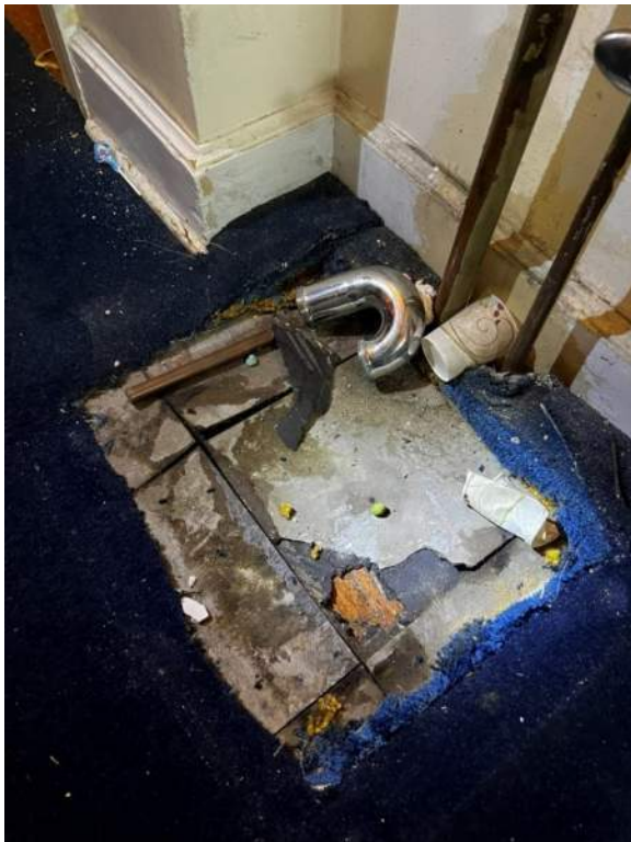
Photo 42: IMG_1241 - Interior 1 st Floor West side hallway to West emergency exit – Water fountains have been removed. Evident water damage at area of removal.
