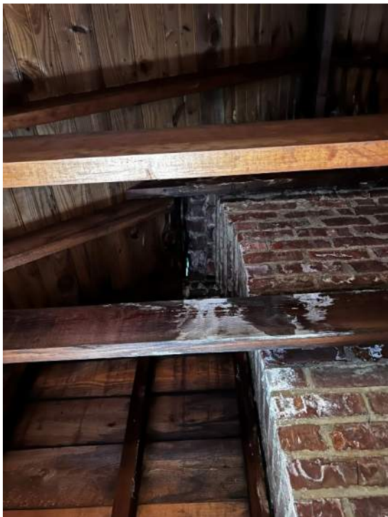
Photo 78: IMG_1575 – East Chimney – Chimney structure is corbelled with significant cantilevered bricks. Visible light between roof framing and chimney representing roof is not fully enclosed for protection from elements. Significant evidence of water infiltration, brick efflorescence on chimney with evident transfer to surrounding wood structure.
