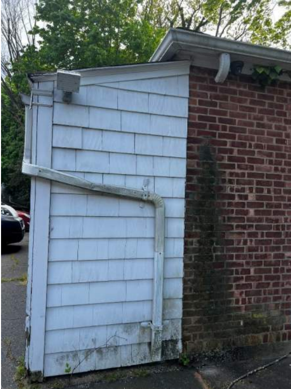
PHOTO 5: IMG_1019 – North Façade : Missing downspout, overgrowth of mold and mildew on façade.
