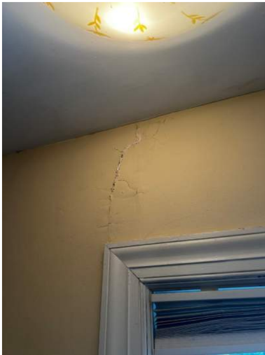
Photo 44: IMG_1427 - East side egress stair, top landing – Moderate cracking in plaster finish with origins from window corners. Requires refinishing (photo 44).
