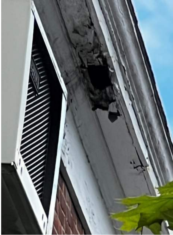
PHOTO 23: IMG_1313 – Missing downspout, significant deterioration of wood fascia, rake boards and soffit.
