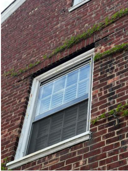
PHOTO 11: IMG_1077 – East Façade – Close up of brick bulging above window headers. Visible shutter brackets with missing shutters.
