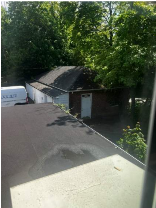
Photo 68: IMG_1517 – Flat roof over rear – exhibits significant ponding on Northwest corner of roof; aligning with deteriorated wall and ceiling of Prep Room below.
