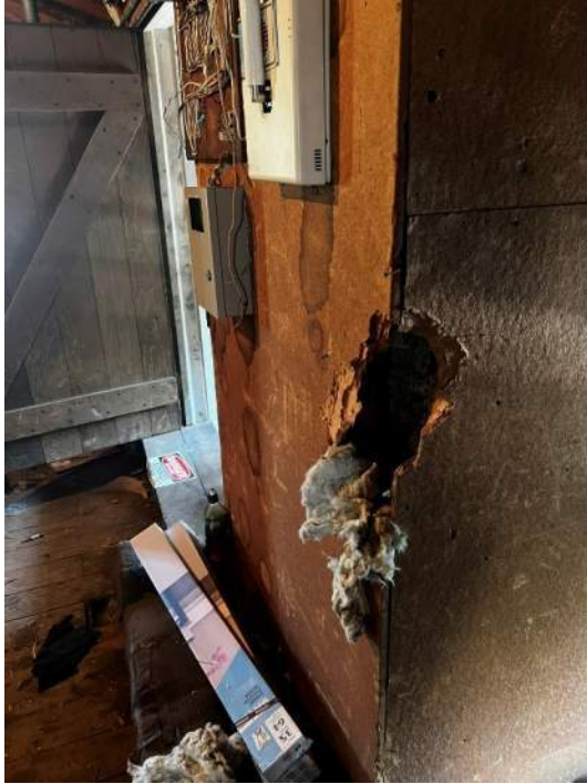
Photo 83: IMG_1622 – Elevator shaft way through attic is constructed of non-rated particle board. Per 2020 BCNYS shaft enclosures shall have a fire-resistance rating of not less than 2-hours where connecting four or more stories. This shaft enclosure connects 4-stories (basement, first floor, second floor and attic) (photo 82).
