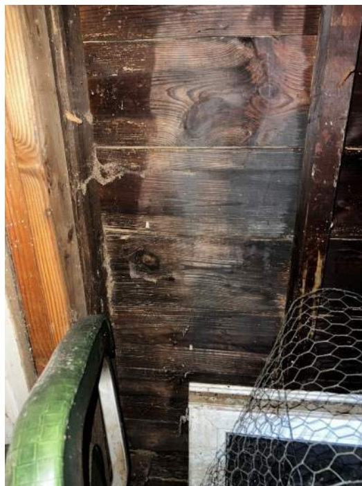
PHOTO 2: IMG_1056 Visible Termite Damage – termite tunnels and droppings
