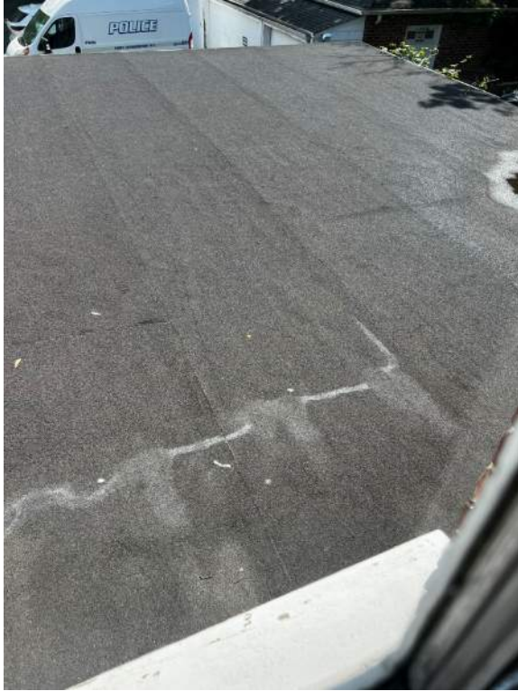
Photo 69: IMG_1518 – Flat roof over rear – Visible efflorescence staining and watermarks on roof surface.
