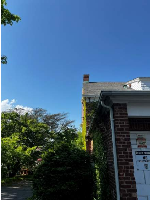
PHOTO 21: IMG_1719 – West Facade–Chimney leaning inwards towards building.
