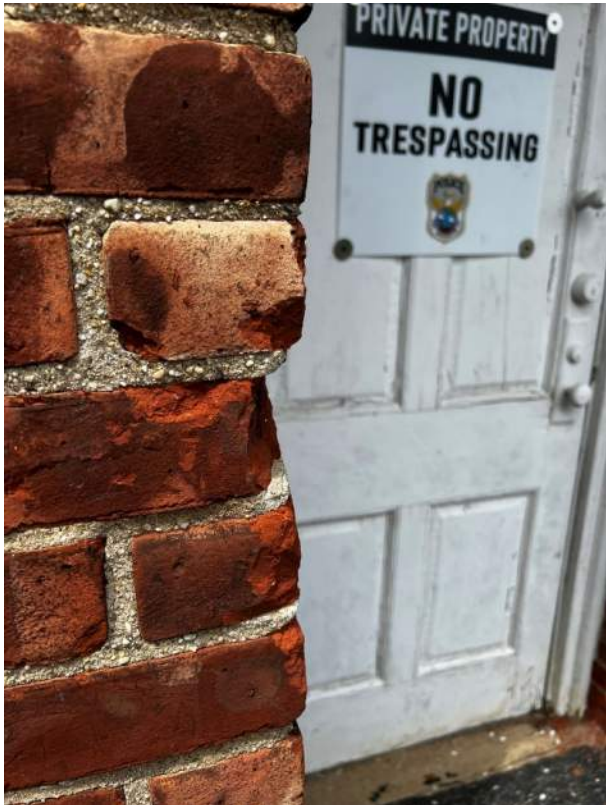
PHOTO 4: IMG_1092 – South East Corner – visible damage to brick masonry
