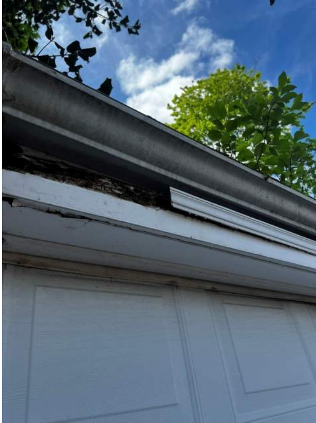
PHOTO 11: IMG_1077 – North Façade. Missing trim work, exposed and deteriorated wood structure.
