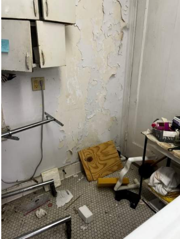
Photo 29: IMG_1183 - Interior 1 st Floor, North West corner of Prep Room – significant water damage for full height of interior corner and ceiling.
