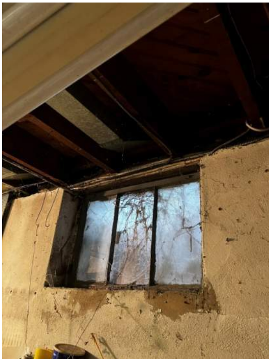
Photo 96: IMG_1302– Visible moisture infiltration at sub-grade windows. Foundation wall paint finish exhibits cracking and chipping. Basement Window wells contain overgrown shrubs and leaves, recommended cleaning of window wells to assess conditions of window frames from exterior.
