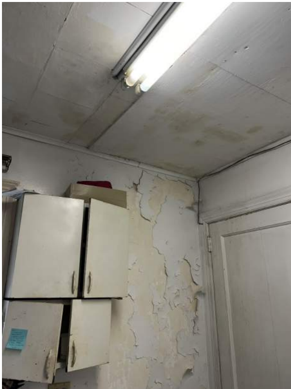
Photo 30: IMG_1182 - Interior 1 st Floor, Northwest corner of Prep Room – significant water damage for full height of interior corner and ceiling.
