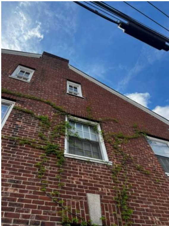
PHOTO 10: IMG_1131 – East Façade – Visible bulging of brick window headers (above lintels), refer to photo 82 for visible water damage at attic window headers.
