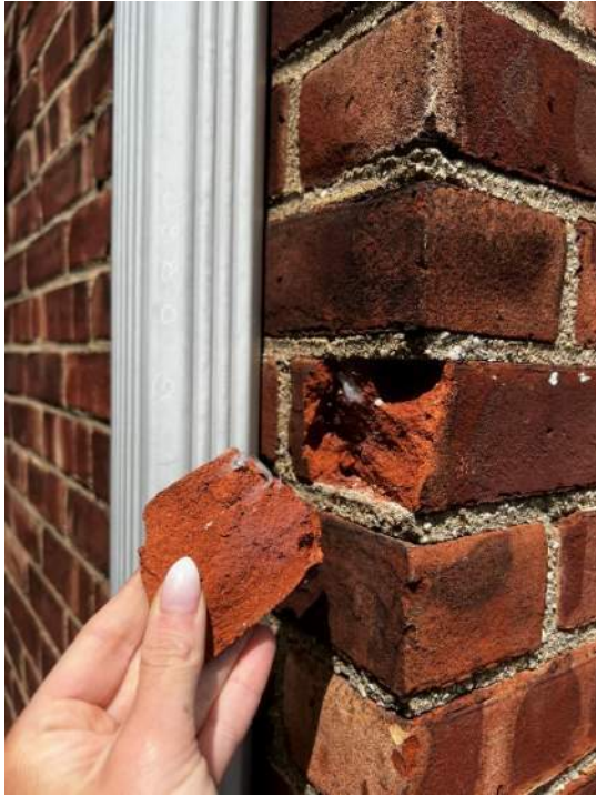
PHOTO 1: IMG_1096 South East Corner – Damage from brick spalling and moisture infiltration
