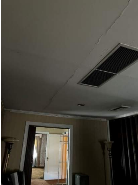
Photo 63: IMG_1489 – Second Floor Northwest Chapel – Ceiling exhibits cracking due to deflection of wood framing. Cracks in ceiling run full length and width of room. Building does not contain emergency egress lights; main source of illumination is portable lamps.
