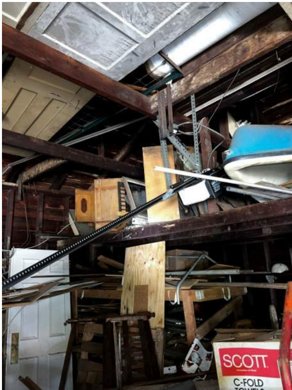
PHOTO 12: IMG_1049 – South Garage door opener / track is broken, requires replacement.
