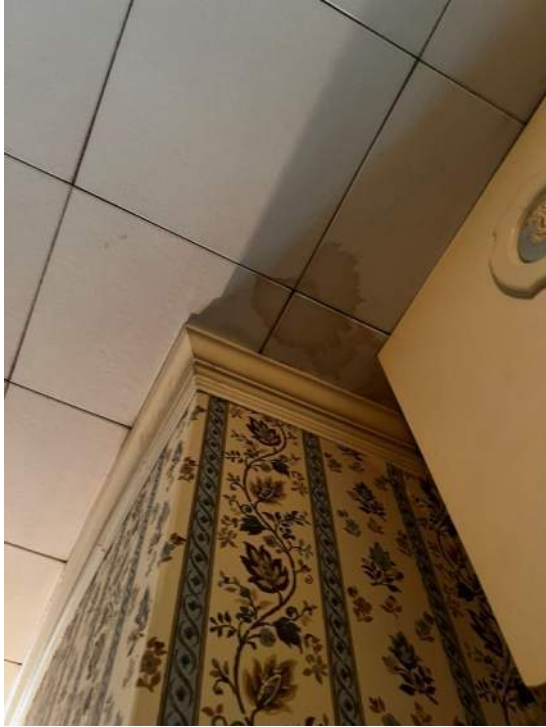
Photo 59: IMG_1475 – Second Floor East Chapel – Leaks evident at ceiling on both sides of the chimney enclosure.
