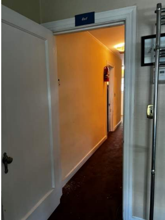
Photo 61: IMG_1487 – Second Floor North Anteroom – Non-compliant illuminated directional exit signage. Non-compliant door hardware for ADA compliance. Fire extinguisher is not mounted in compliance with NFPA 10. If mounted in compliance with NFPA 10, fire extinguisher would be non-compliant with ADA for protruding objects and would reduce the minimum required clear width of the hallway.
