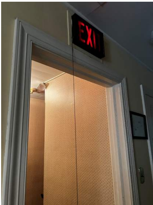
Photo 52: IMG_1444 – Second Floor Corridor – Emergency exit sign is present, but not continuously illuminated. Pull string cord activates illumination. Exit sign is not directional.
