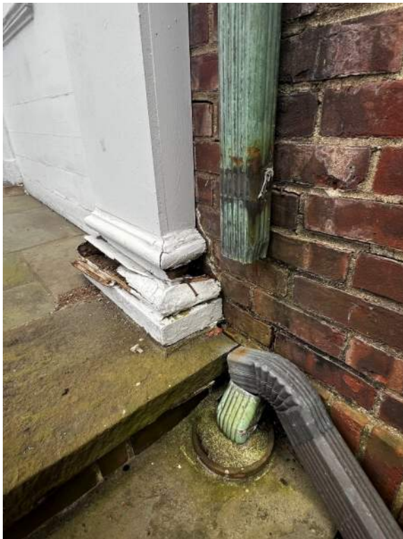
PHOTO 18: IMG_1327 – North Façade (North West of front entrance) - Internal downspout to collector box is dislodged, allowing water to drain onto brick masonry and wooden elements. Significant deterioration of wooden pilasters and trim at front entry.
